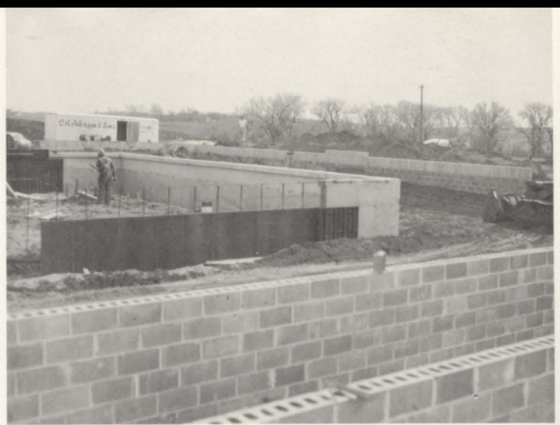
Construction is well underway on the new West Sioux High School.
