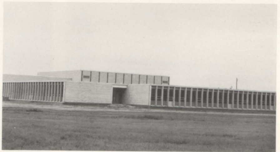
The new West Sioux High School will be completed this summer and ready for students this fall.
