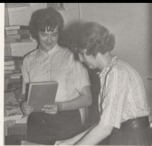
Lois Moeller and Janice Schlueter pack library books in preparation for the move to the new building.
